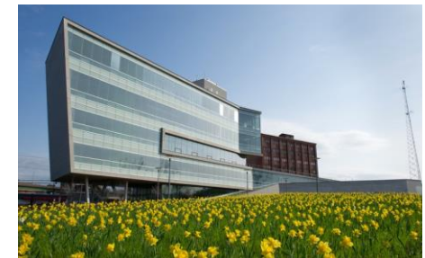
b. Whole Building Testing at SyracuseCOE
